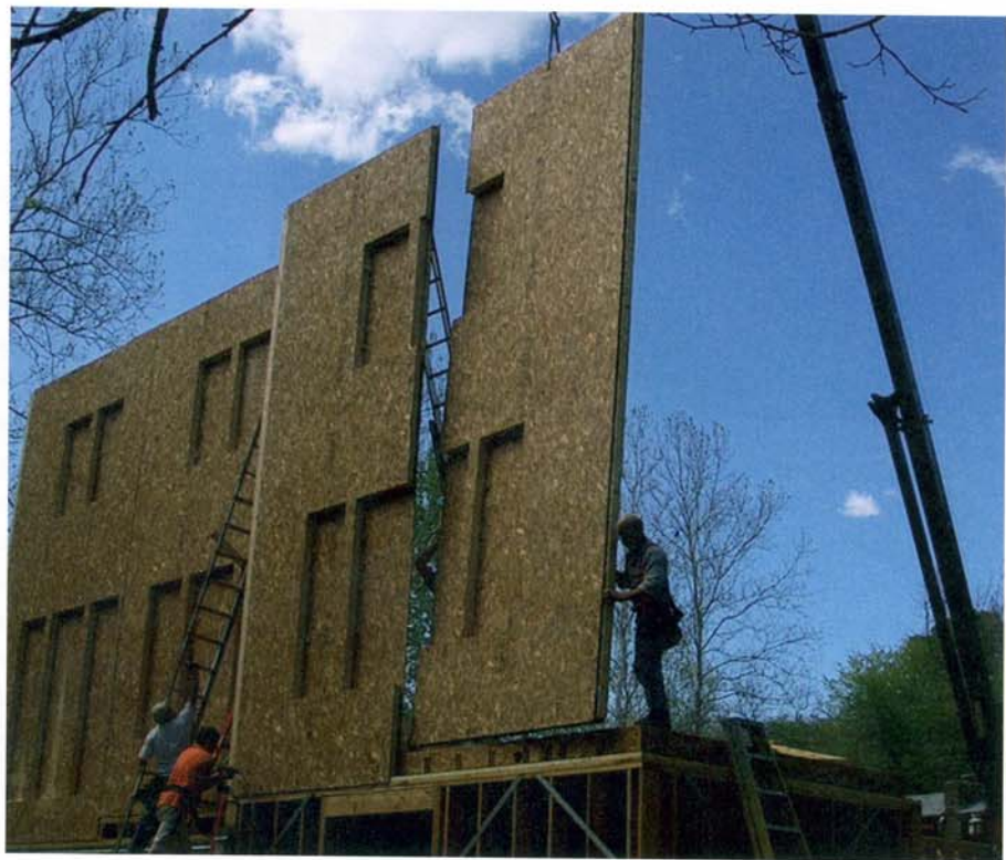
Left: Husband and wife team Rick Robson and Kelly Parker did a considerable amount of the construction and finish work on their eco-friendly home in Parkville. Right: The shell of the house was erected in 10 hours using structural insulated panels (SIPs), which provide a high insulation factor in the walls and roof.
