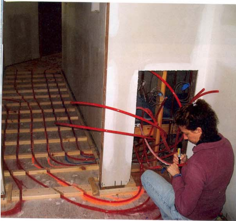
Top: The outside of the house is primarily covered in HardyPlank fiber cement-based siding that is eco-friendly because of its durability and resistance to water damage. Middle: Homeowner Kelly Parker worked on the radiant floor heating system, creating a second-floor heating zone that allows the couple to better control their energy usage. Bottom: Homeowner Rick Robson used a chain saw to craft a unique fireplace mantle from a walnut tree that had died on the property.
