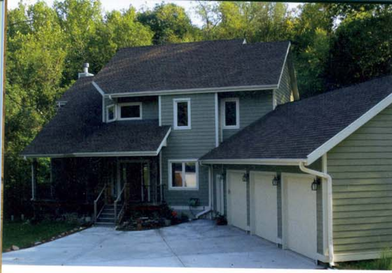
Top: The outside of the house is primarily covered in HardyPlank fiber cement-based siding that is eco-friendly because of its durability and resistance to water damage. Middle: Homeowner Kelly Parker worked on the radiant floor heating system, creating a second-floor heating zone that allows the couple to better control their energy usage. Bottom: Homeowner Rick Robson used a chain saw to craft a unique fireplace mantle from a walnut tree that had died on the property.
